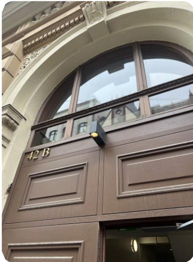
1. The accessible entrance at Aleksanterinkatu
