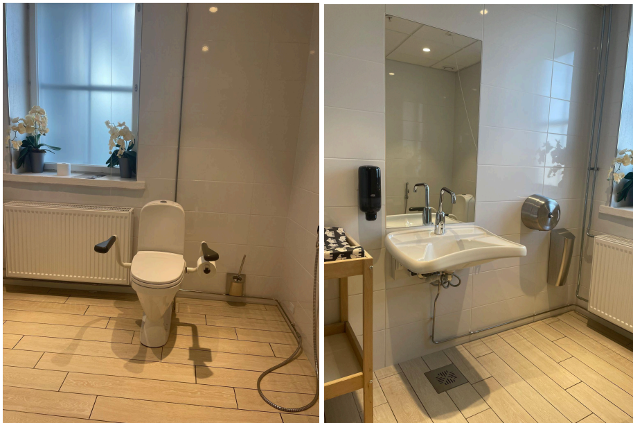
Accessible toilet 2 (on the second floor):
